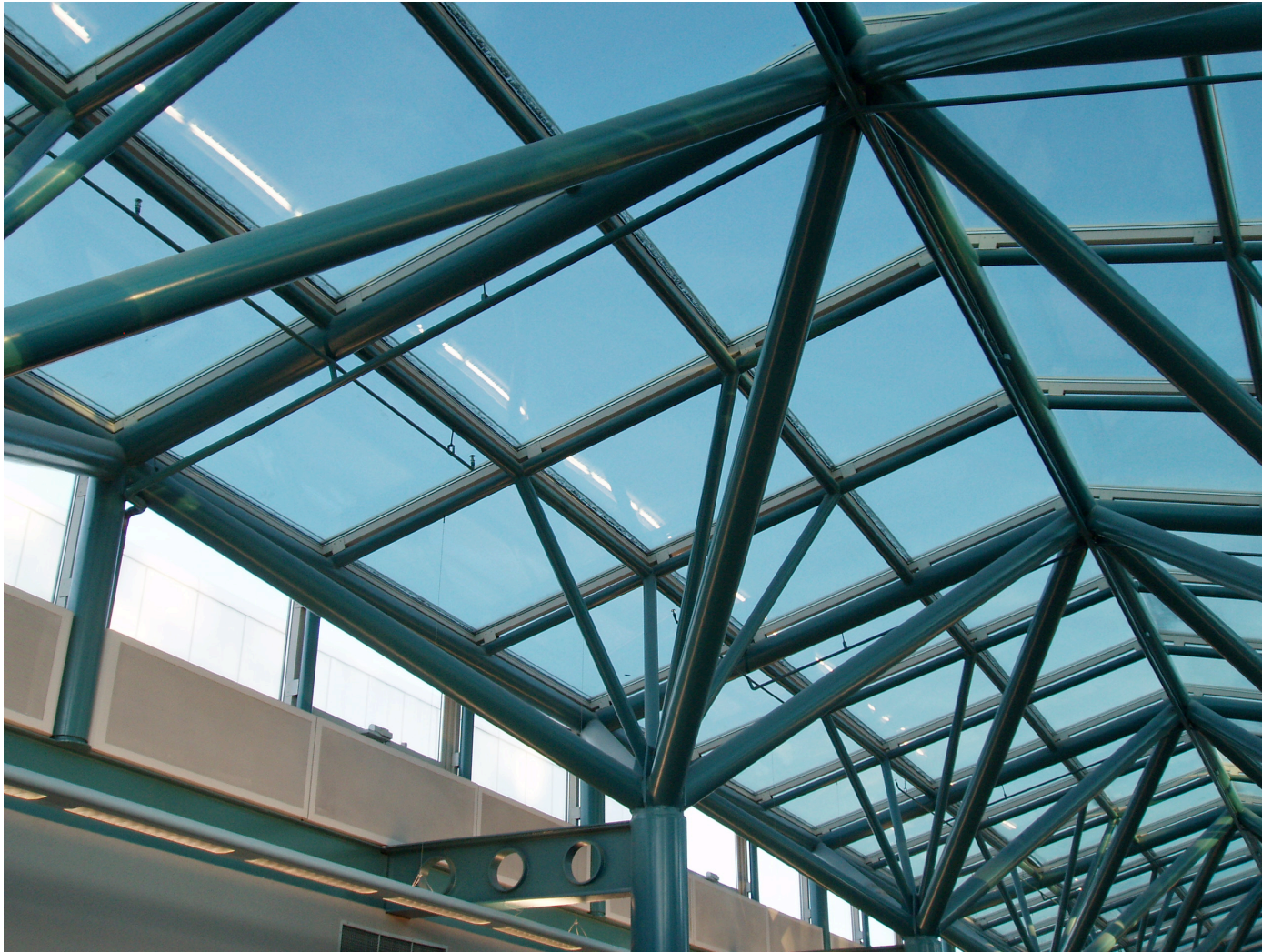
Applied Science Building, Simon Fraser University, Burnaby.
