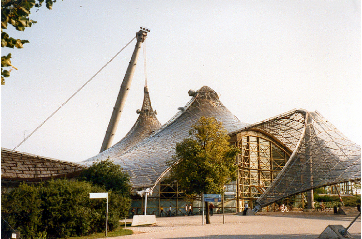
Partial view of the hyperbolic roof Olympiapark, Munich, tensile structure
